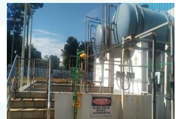
Bund for Hazardous Chemical
